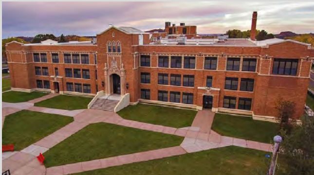
Buildings like the Luther L Wright School shape the historic character of Ironwood.
