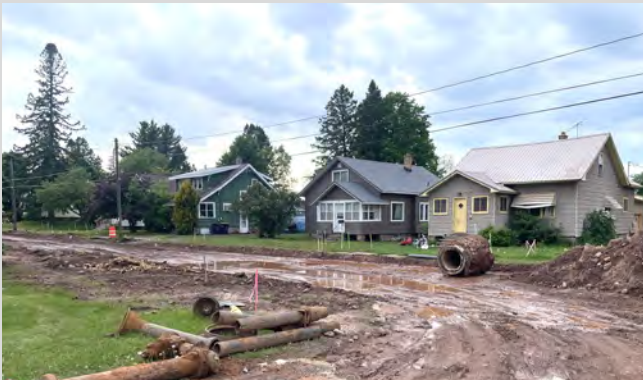
Ongoing improvements to replace aging pipes
