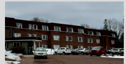
Existing higher density housing in Ironwood
