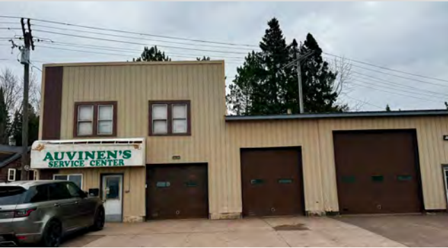
Existing uses in the Business Development District include small auto repair.
