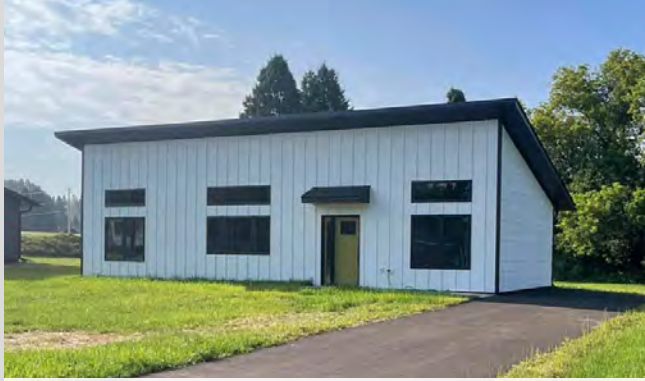
New construction on a vacant lot in Ironwood.
