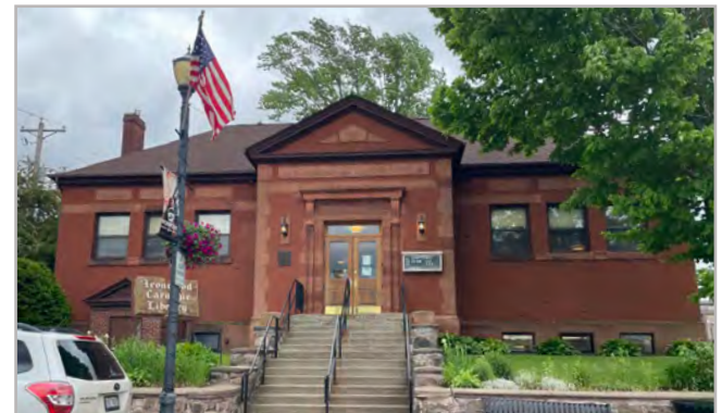
Public Facility - Library
