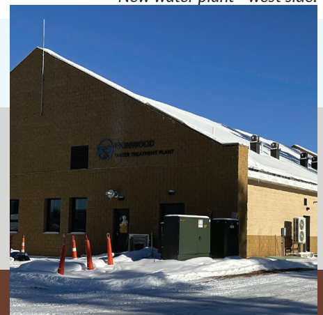
New water plant - west side.
