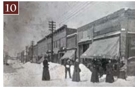
10 Lieberthal Block - corner of S. Suffolk and E. McLeod Ave. ca. 1899
